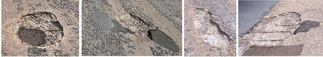
***Figure 4.4. The surface condition highlights prevalent issues such as potholes and damaged surfaces. Potholes and surface damage can disrupt the impactor's contact with the bridge, leading to variations in the generated mechanical waves.***
