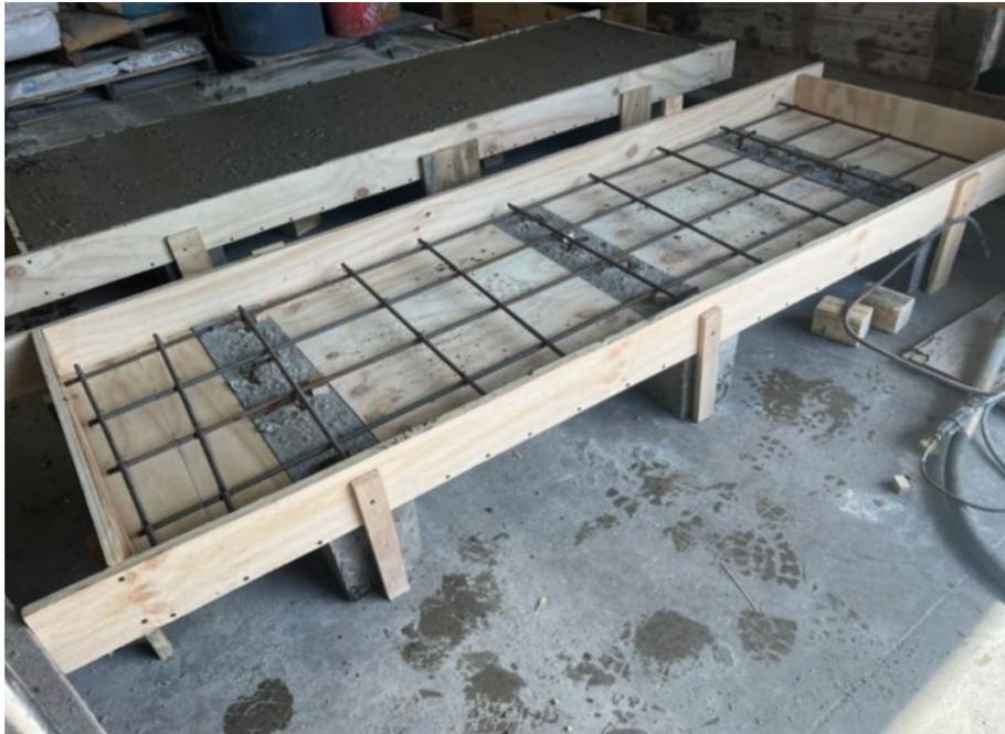
Figure 4 - 14 Concrete Decks Formworks and Casting
