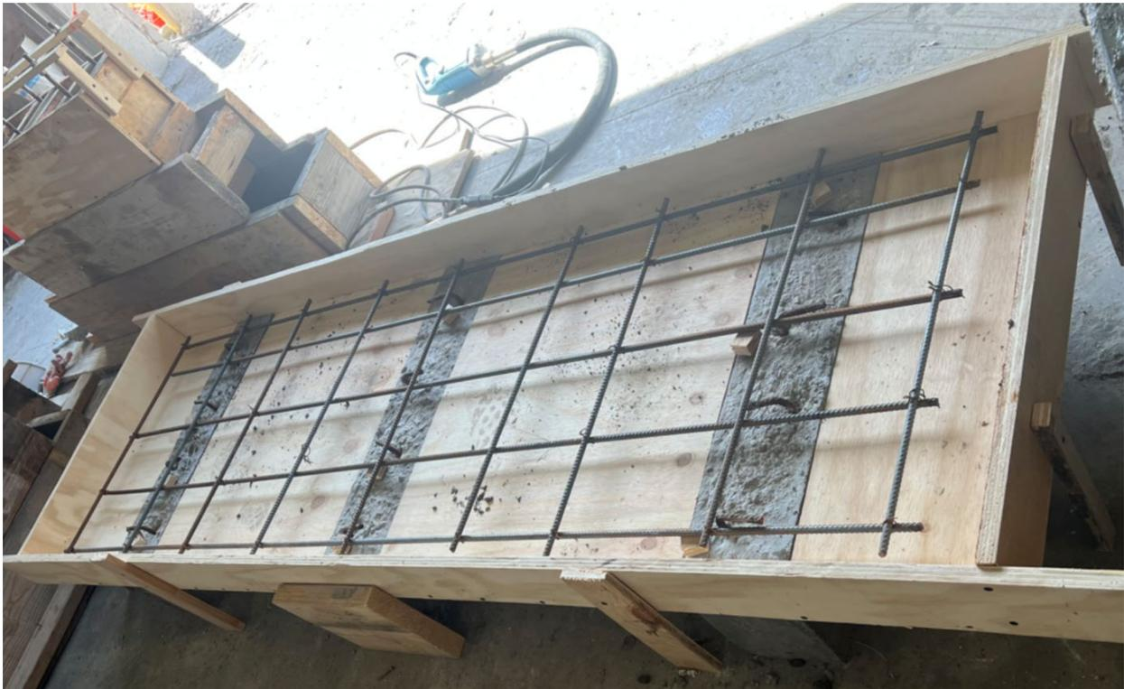
Figure 4 - 5 Formworks and Bottom Layer Reinforcement of AASHTO LRFD Concrete Deck
