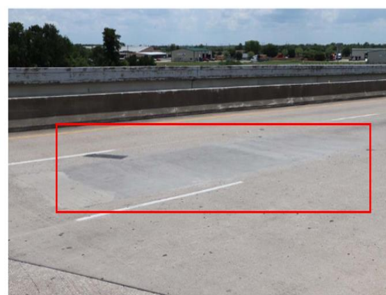
Figure 1-5 Failure patterns in span 2 of EB bridge (TxDOT): (a) CIP deck; (b) PCPs
