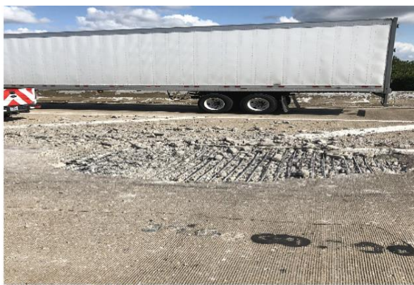
Figure 1-5 Failure patterns in span 2 of EB bridge (TxDOT): (a) CIP deck; (b) PCPs
