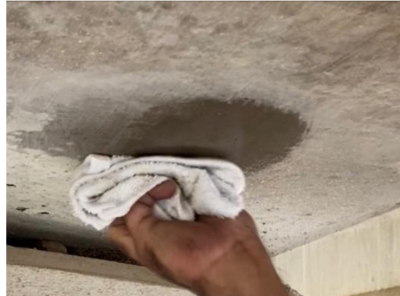
(b) Cleaning surface with acetone
