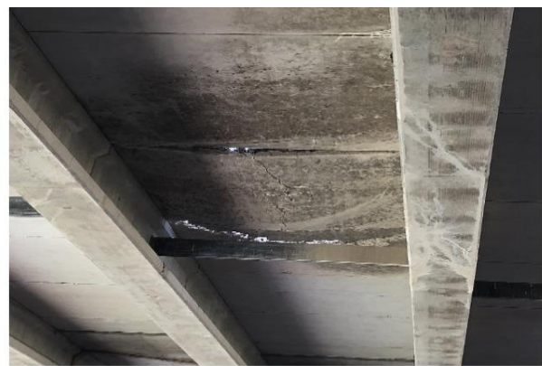
Figure 1-5 Failure patterns in span 2 of EB bridge (TxDOT): (a) CIP deck; (b) PCPs
