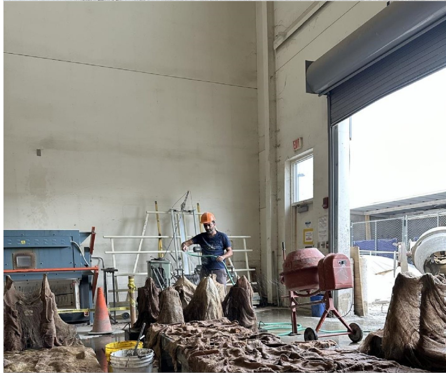
Figure 3.20 SFRC During the Pouring Day and After
