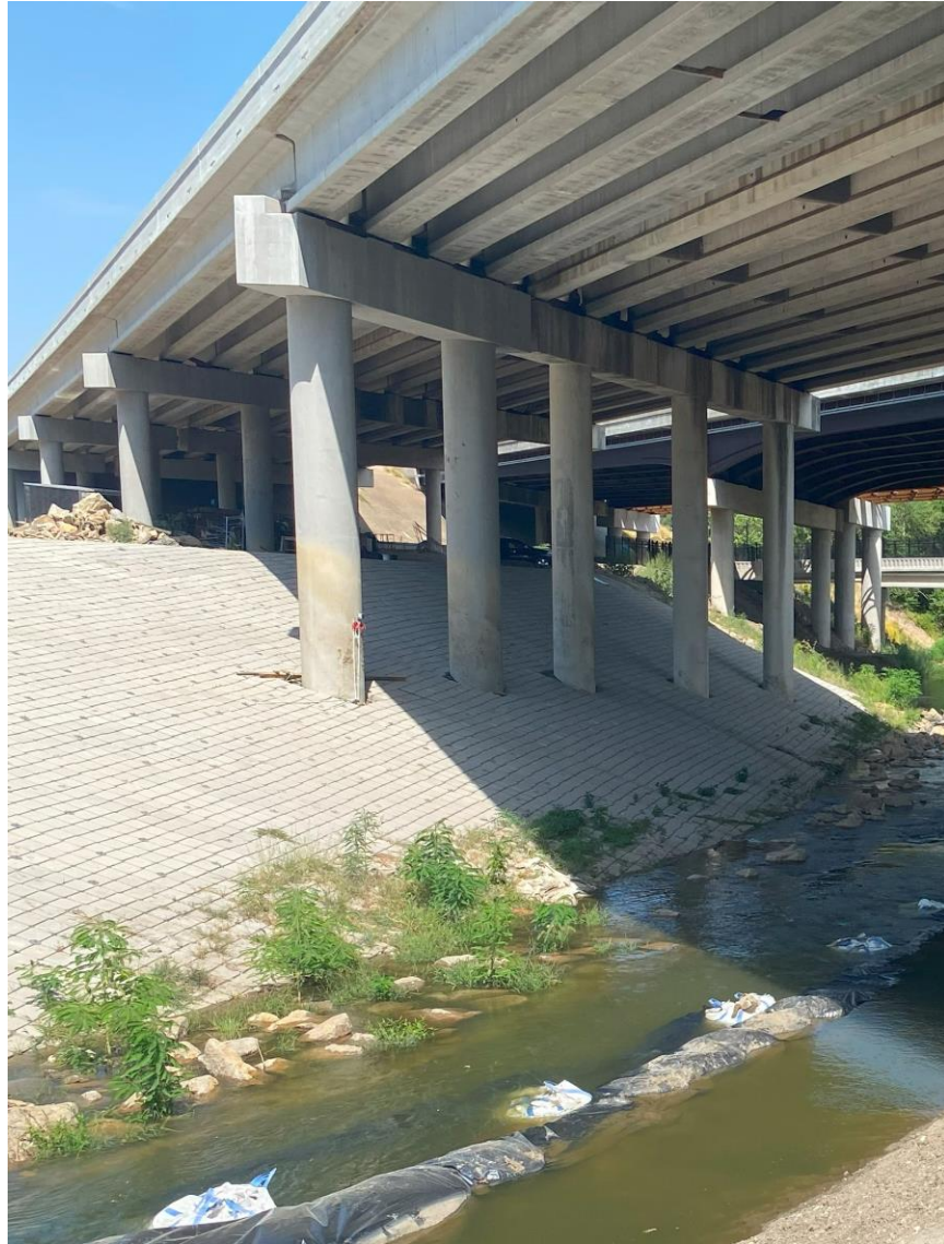
Figure 35- IH-20 project's slope after stabilization.
