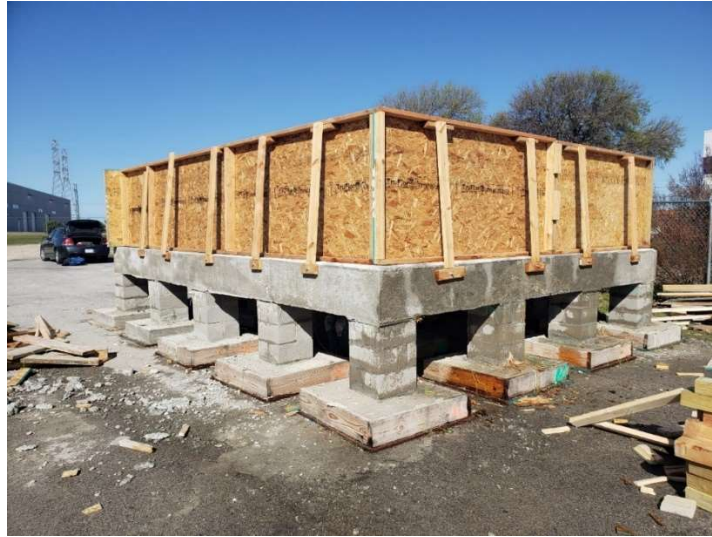
Figure 12: Waterproof Basin Constructed on Top of Slab
