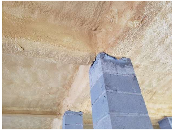
(b) Elevated Slab with Steel Beam Supports (c) New Pier under Existing Grade Beam
