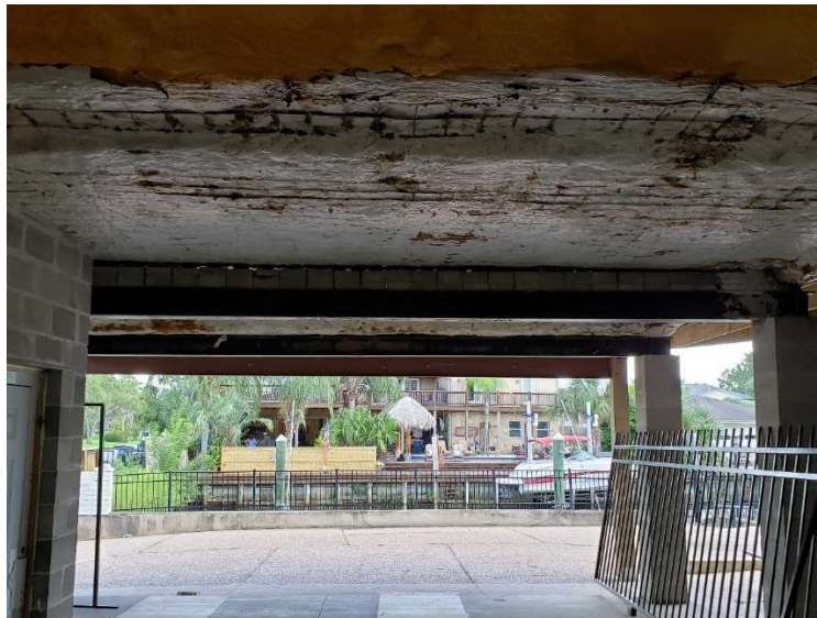
Figure 4: Elevated Home Supported by CMUs and Steel Beams
