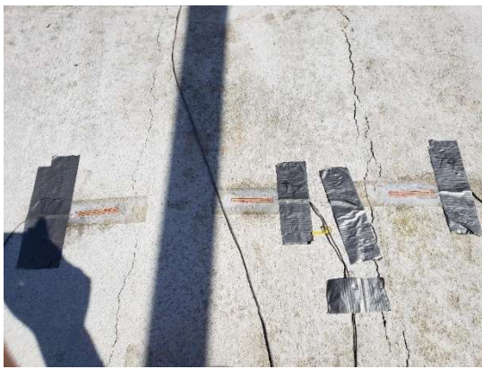
(a) Top Surface of Four-Panel Slab
