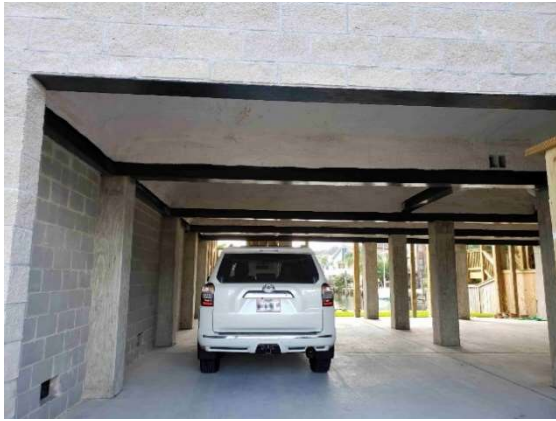
(b) Elevated Slab with Steel Beam Supports (c) New Pier under Existing Grade Beam
