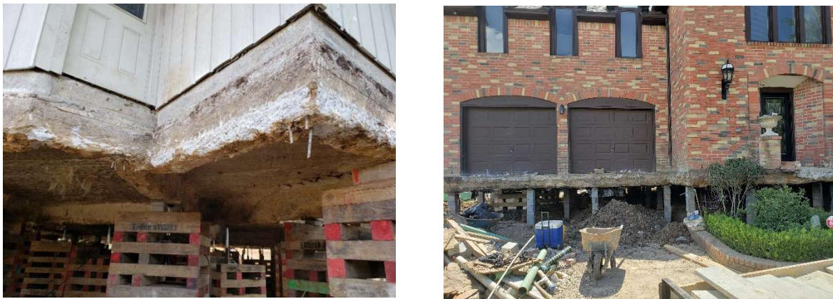
(a) Homes in the Process of Being Elevated
