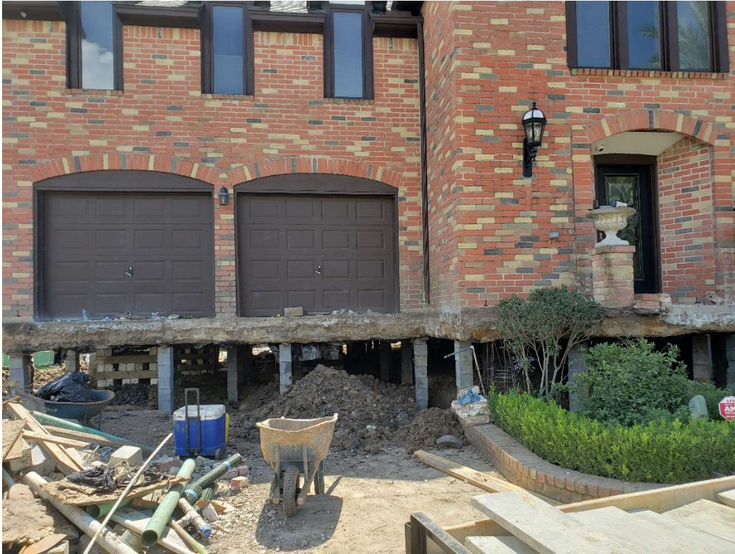
Figure 3: Nassau Bay Home in the Process of Being Elevated
