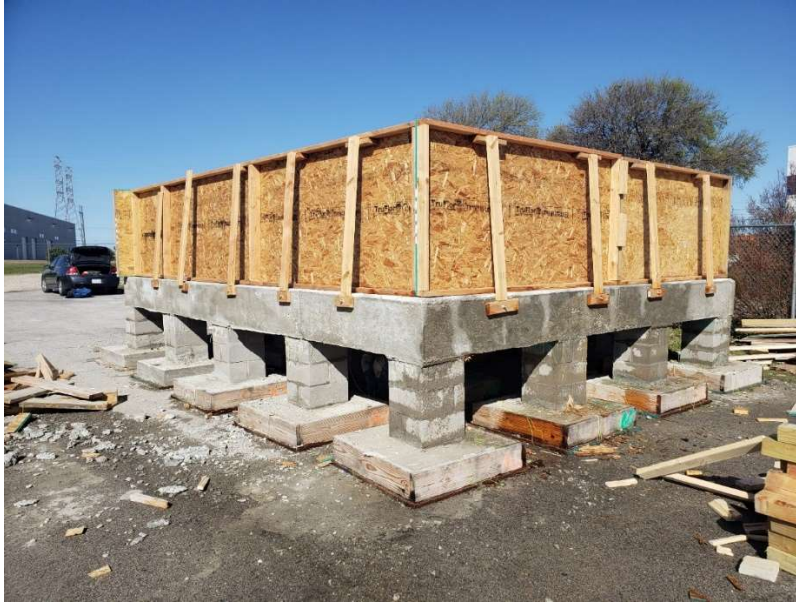
Figure 25: Experimental Elevated Slab Specimen
