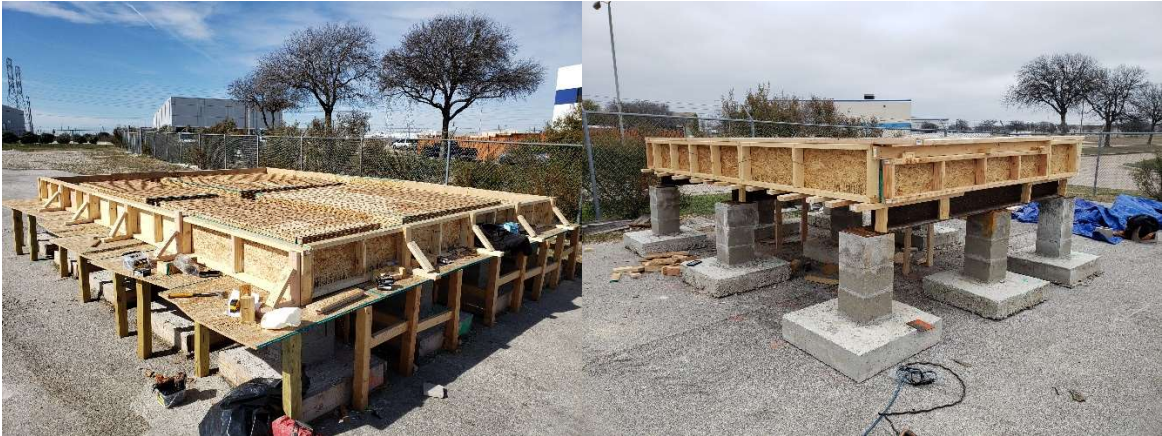
b) Slab Formwork Assembly
