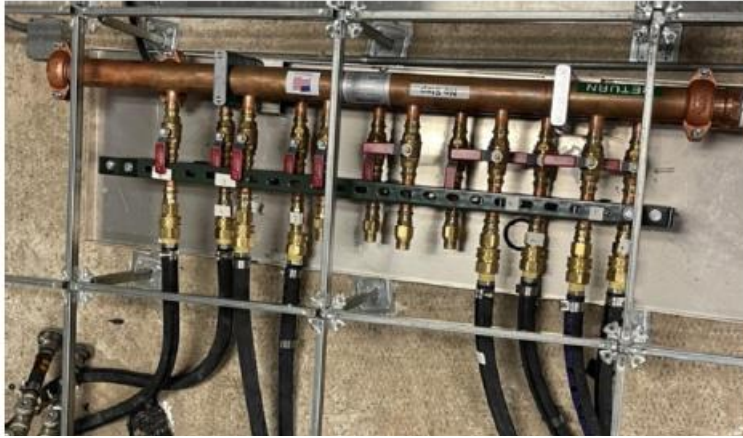
FIGURE 4.2: ROW MANIFOLD
