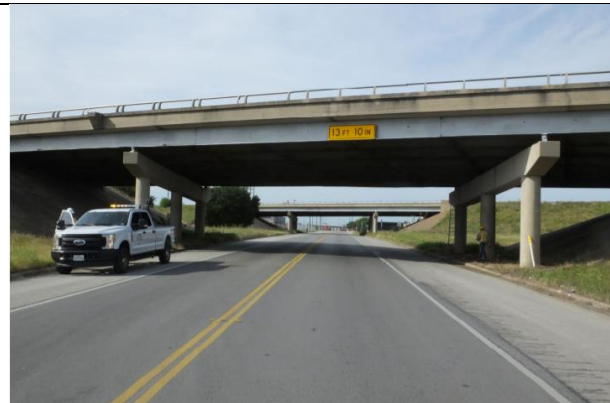
Roadway Under Carey St. Looking West
