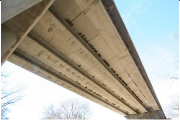
SUPERSTRUCTURE Looking Southwest
