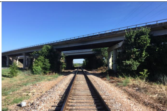
Railroad Under Bridge (Looking Northwest)
