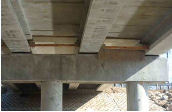
Timber bracing/forms left in place at east bent
