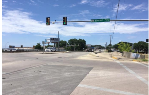
ROADWAY OVER BRIDGE - SYLVANIA AVENUE NORTHBOUND (LOOKING NORTH)
