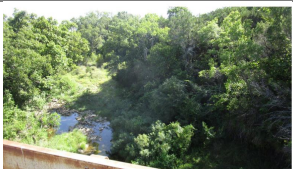
8 - Downstream looking Northeast
