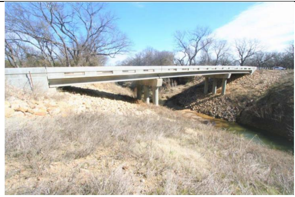
ELEVATION Looking Northeast
