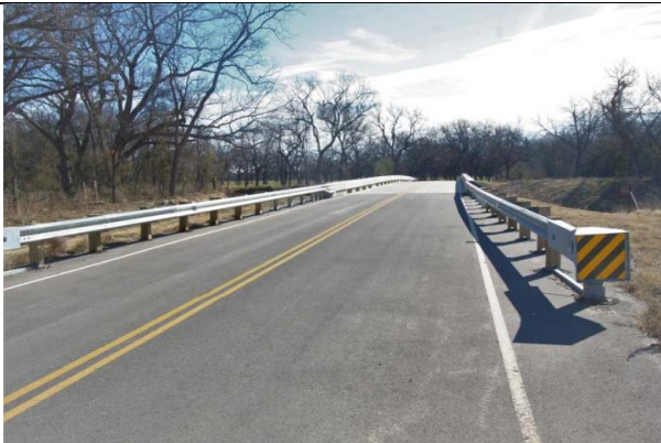
ROADWAY OVER BRIDGE Looking East
