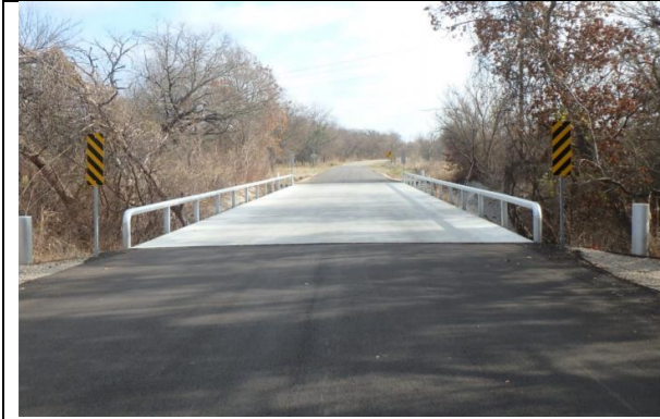
ROAD OVER LOOKING SE
