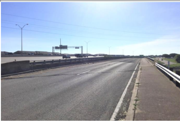
Roadway Over Bridge (Looking East)
