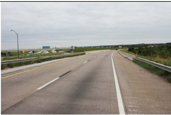
Roadway Ih 20 Eb Looking Southeast
