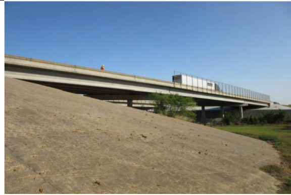
Elevation Up Rr Looking Northeast
