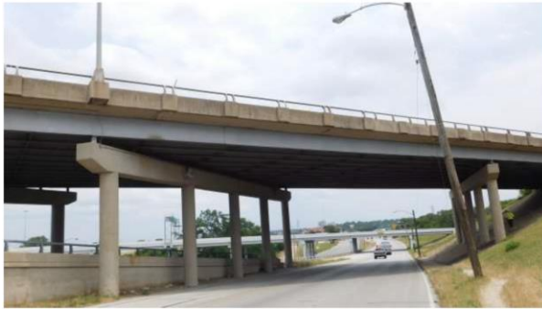
Roadway Under Looking East
