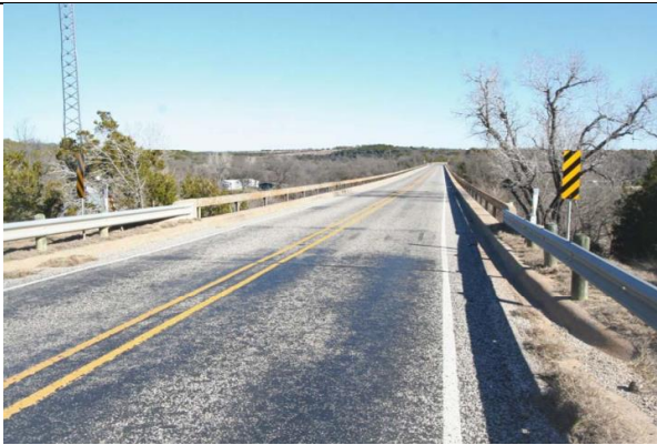
ROADWAY OVER BRIDGE Looking North
