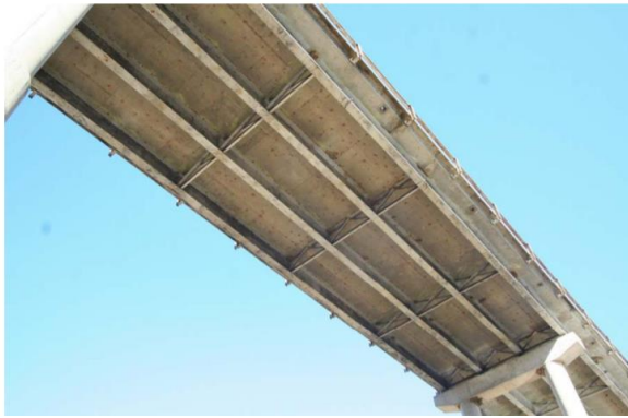
SUPERSTRUCTURE Looking Northwest
