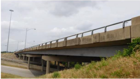
Elevation Looking Southwest
