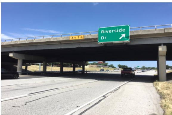
ROADWAY UNDER BRIDGE - SH 121 NORTHBOUND (LOOKING EAST)
