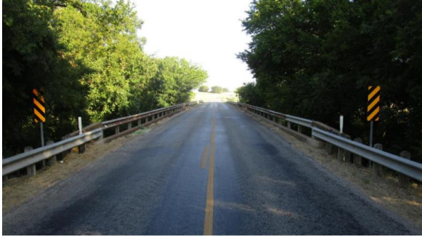
1 - Roadway looking Northwest (FM 2156)
