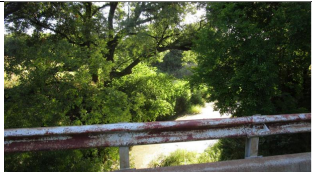
6 - Upstream looking Northeast
