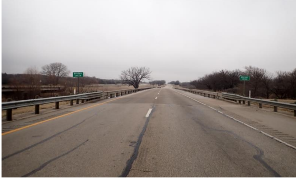
Roadway View Looking Northwest.
