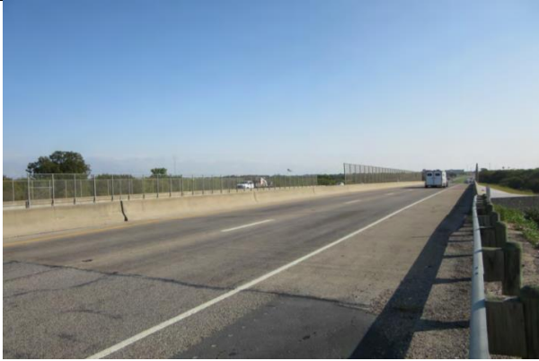
Roadway View Us 67 Nb Looking East
