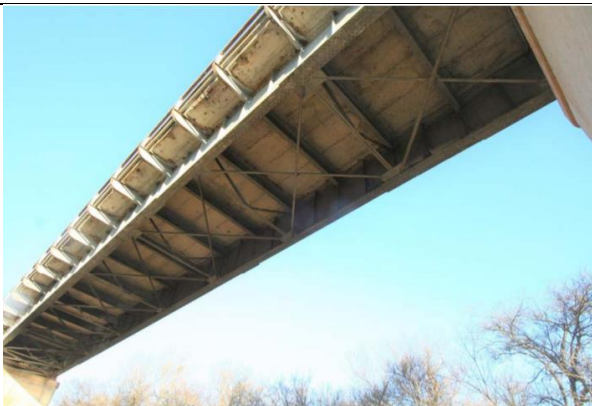
SUPERSTRUCTURE Looking Northwest
