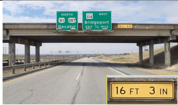
Roadway (Us 81/287 Wb) Under View in Span 2 Looking West
