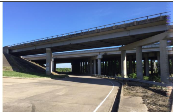
Roadway Under Bridge - West Turnaround (Looking Northwest)
