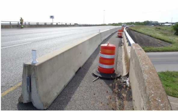
Closed W. Shoulder Looking South
