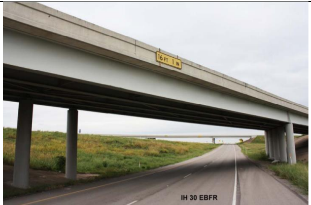
IH 30 EBFR 16 FT 1 IN LOOKING EAST
