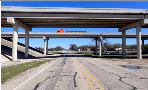
Roadway (FM 730) under view in Span 2 looking south.
