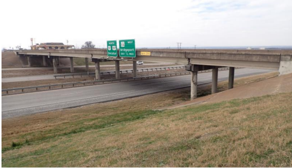
East Bridge Elevation Looking Southwest.
