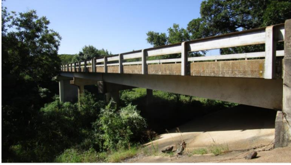
3 - Elevation looking South
