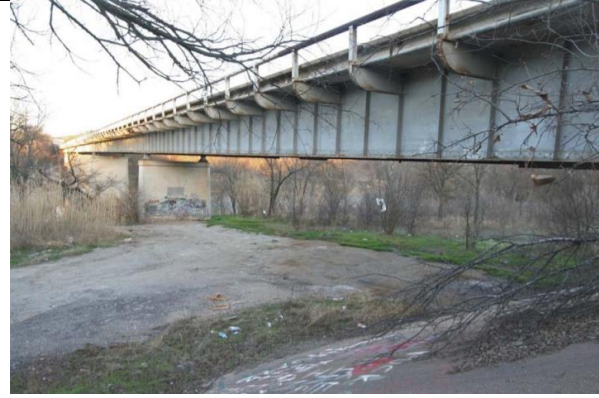
ELEVATION Looking Northwest
