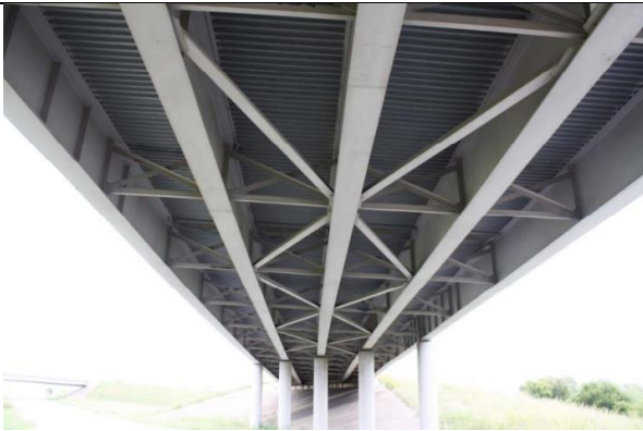
Superstructure Looking Southeast
