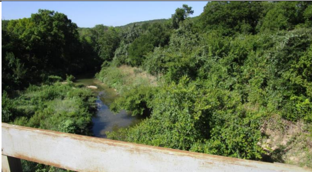
7 - Upstream looking Southwest
