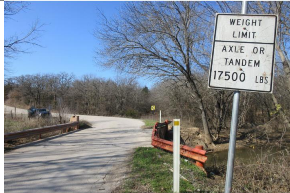
Load Posting - East Approach Looking West
