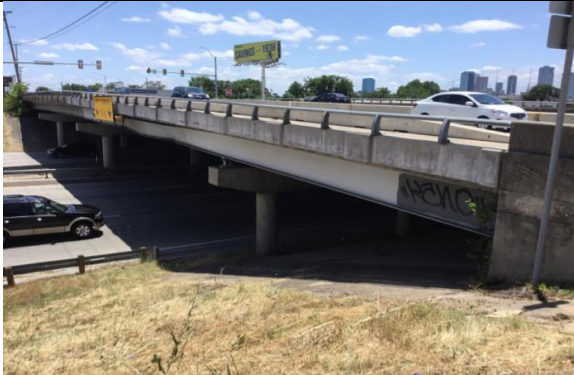
ELEVATION (LOOKING SOUTHWEST)
