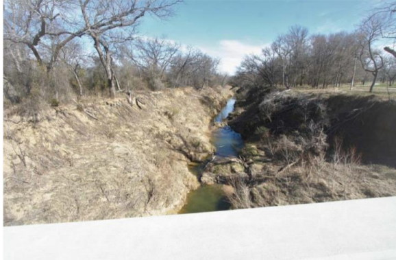
DOWNSTREAM VIEW FROM BRIDGE Looking North
