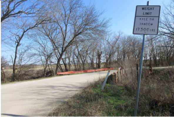
Load Posting - West Approach Looking East
