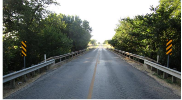
2 - Roadway looking Southeast (FM 2156)
