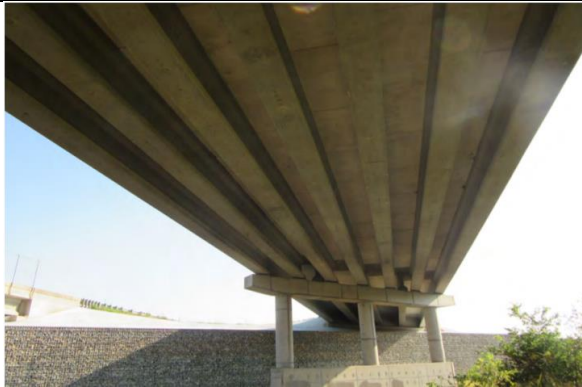
Superstructure Looking East
