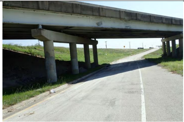
ROADWAY UNDER BRIDGE IH 35W SB EXIT Looking Southeast
