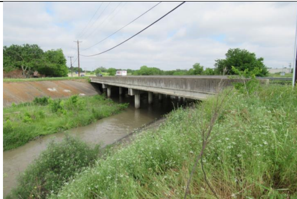
SIDE VIEW Looking Northwest
