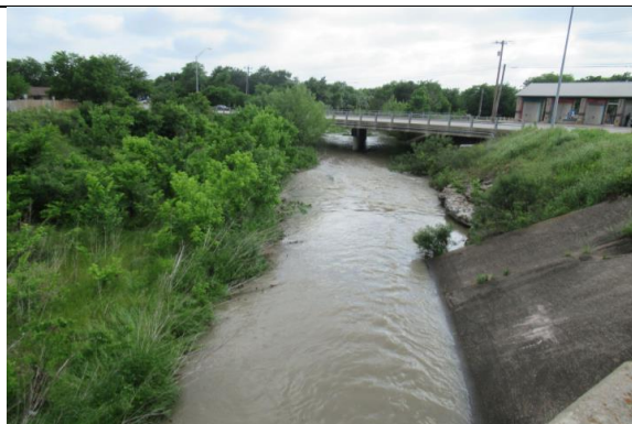
DOWNSTREAM CHANNEL Looking Southeast
