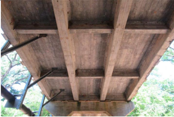
SUPERSTRUCTURE VIEW Looking East
