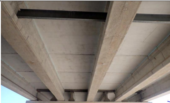
Underside of superstructure in Span 1 looking east.
