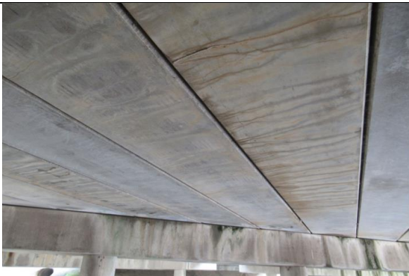
SUPERSTRUCTURE VIEW Looking East
