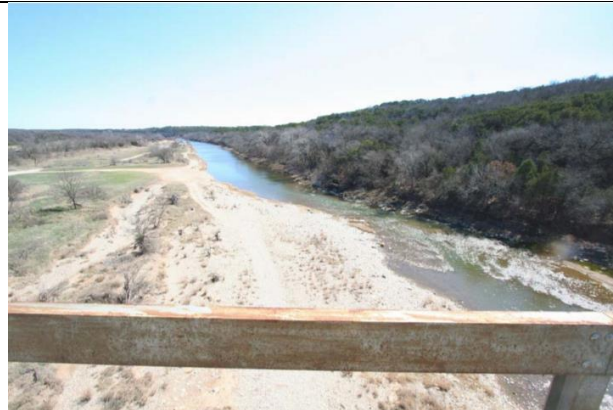
DOWNSTREAM VIEW FROM BRIDGE Looking East
