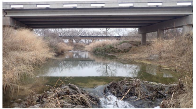
Channel Under View Looking Northeast
