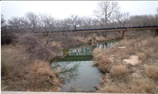
Upstream Channel Looking Northeast
