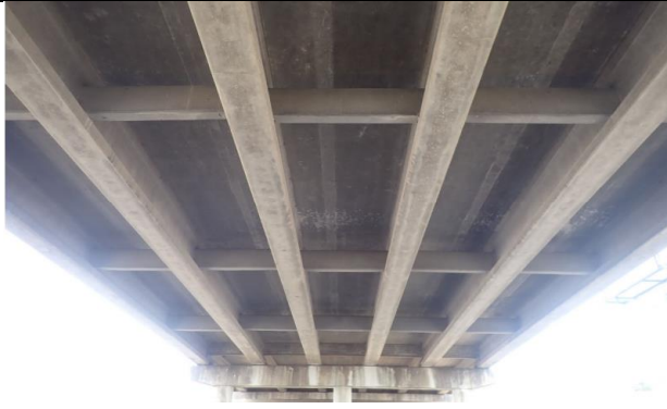
Underside Of Superstructure in Span 2 Looking North.
