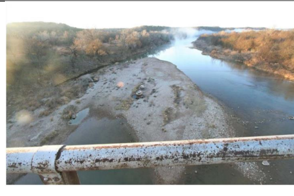
DOWNSTREAM VIEW FROM BRIDGE Looking South
