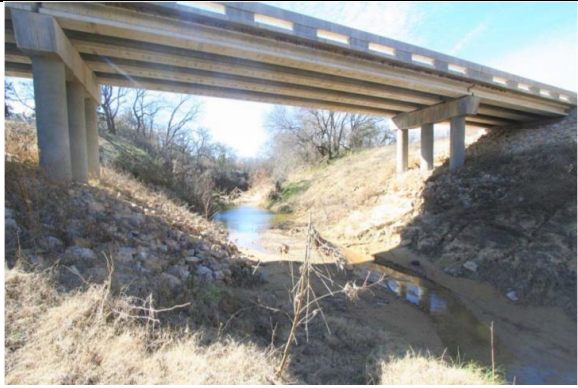
STREAM UNDER BRIDGE Looking South
