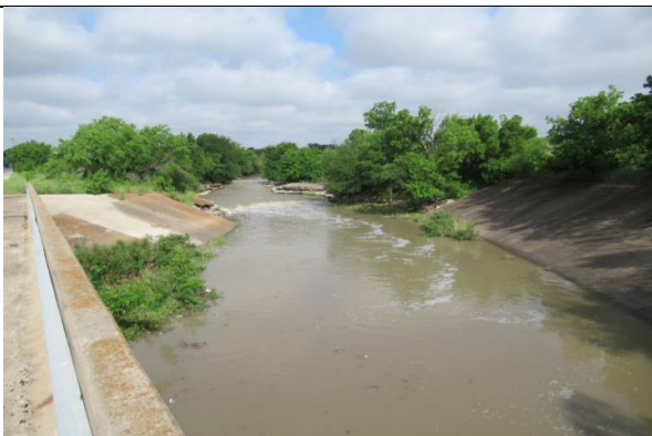
UPSTREAM CHANNEL Looking Northwest
