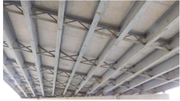
Under Looking South
