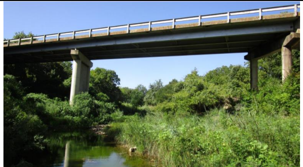
6 - Stream Under looking Southwest
