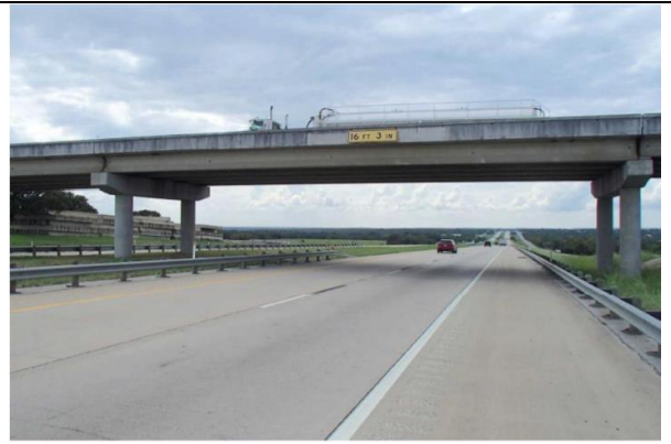
IH 20 WB UNDER Looking West
