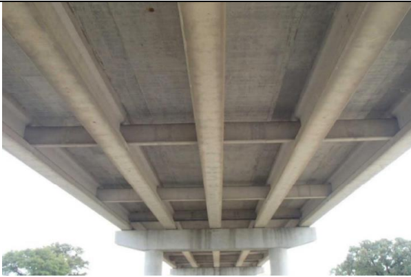
SUPERSTRUCTURE Looking South
