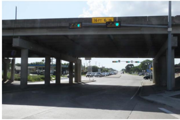
Roadway Under Bus 287 Sb - Looking Southeast
