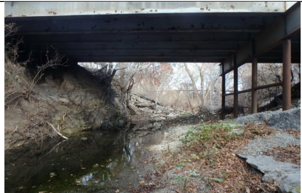
Stream under looking NE
