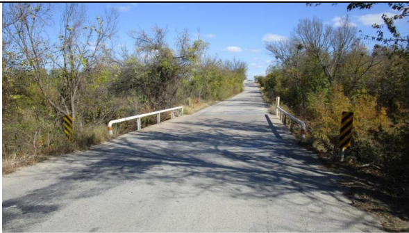
1 - Roadway looking East (CR 915 - PCT. 2)
