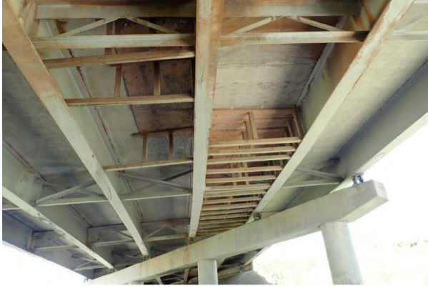
PREVIOUS CONCRETE DECK REPAIRS Looking North
