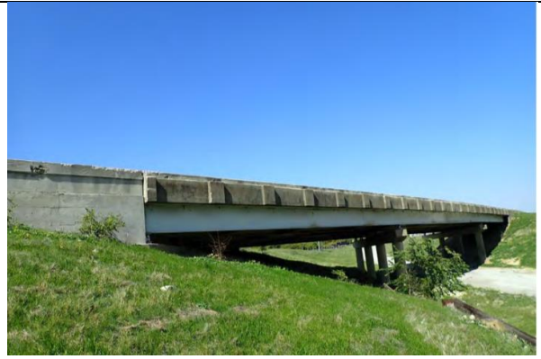
SIDE VIEW Looking Northwest
