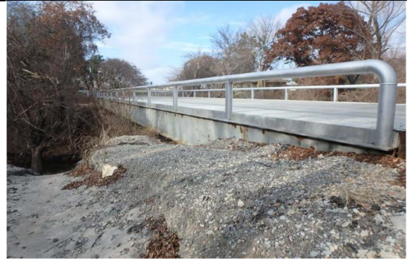
ELEVATION LOOKING NORTH
