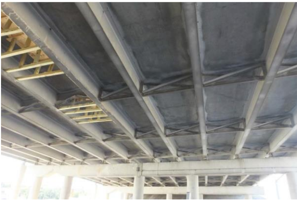
Superstructure - Looking Northeast
