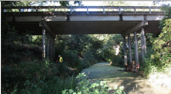
5 - Stream Under looking Southwest
