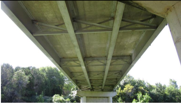
5 - Under looking Southeast
