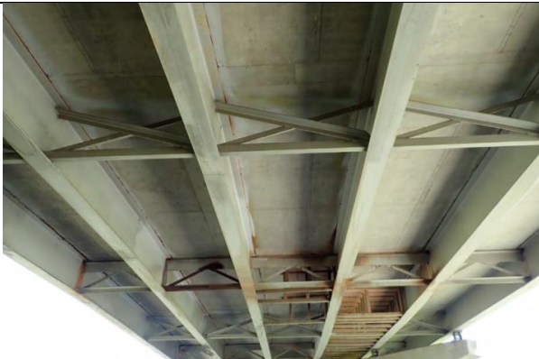
SUPERSTRUCTURE Looking North
