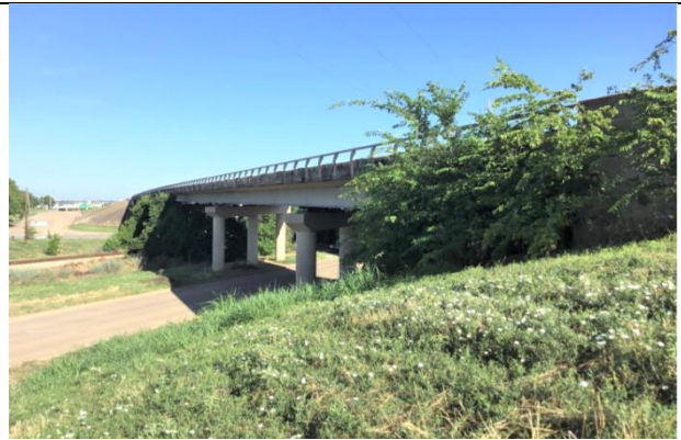
Elevation (Looking West)
