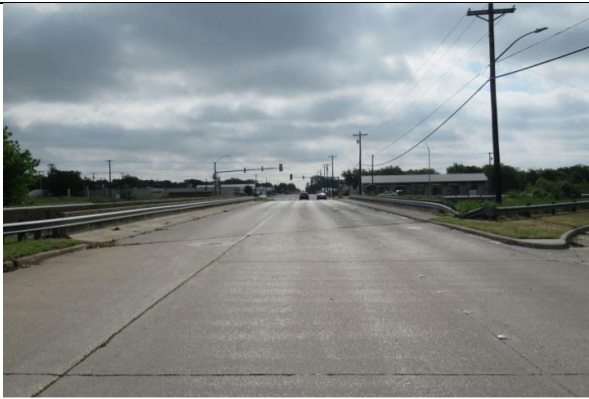
ROADWAY VIEW Looking East
