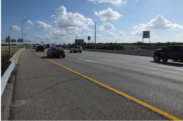
Roadway Over Bridge - Looking Southwest
