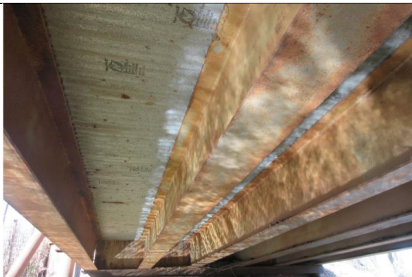
Superstructure View Looking West
