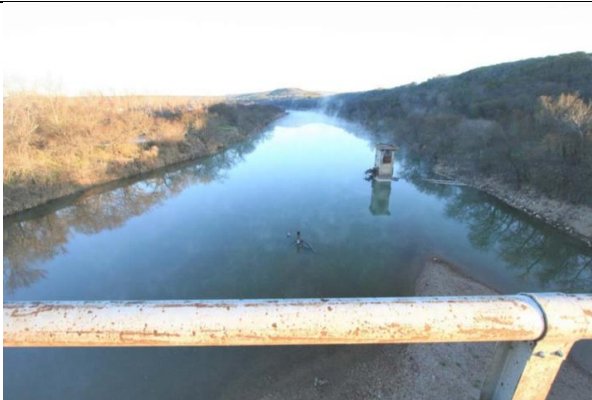
UPSTREAM VIEW FROM BRIDGE Looking North
