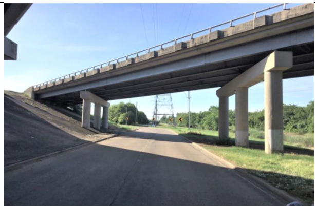
Roadway Under Bridge - East Turnaround (Looking Southeast)
