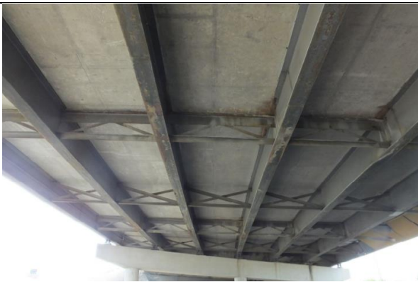
Superstructure Looking South
