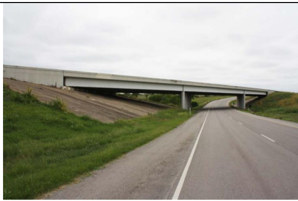
Elevation Ih 30 Ebfr Looking Southwest
