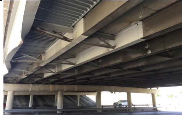
SUPERSTRUCTURE (LOOKING SOUTH)
