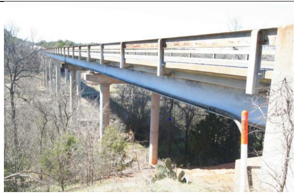
ELEVATION Looking Southwest
