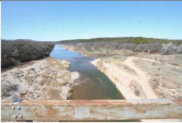
UPSTREAM VIEW FROM BRIDGE Looking West
