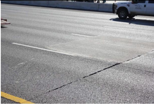
Full Depth Deck Repair NE Span Looking Southwest
