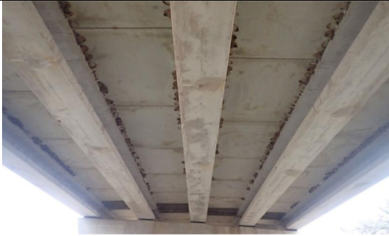
Underside Of Superstructure In Span 2 Looking Northwest.
