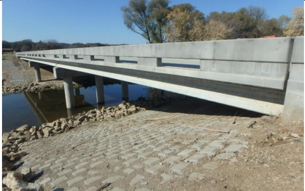
Elevation looking nw
