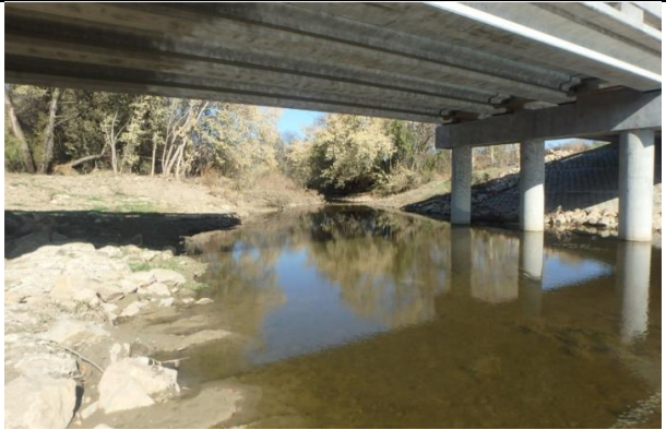
Stream under looking north
