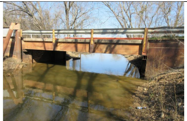
Stream Under Bridge Looking North
