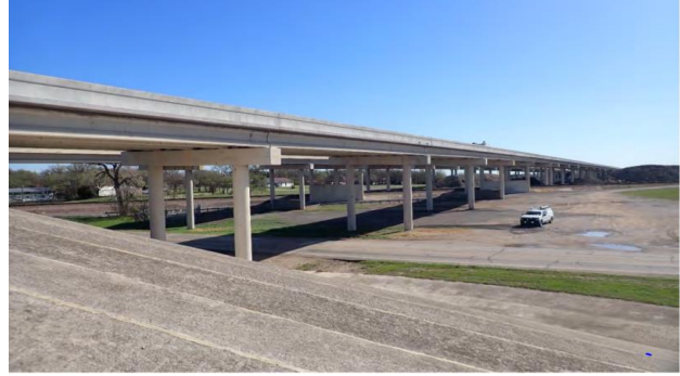
South bridge elevation looking northeast.
