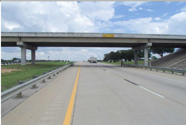
IH 20 EB UNDER Looking East
