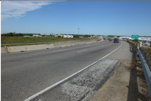
Roadway Over Bridge Looking North
