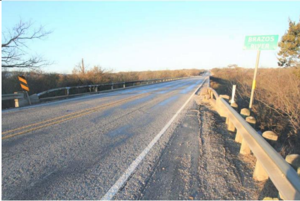
ROADWAY OVER BRIDGE Looking West
