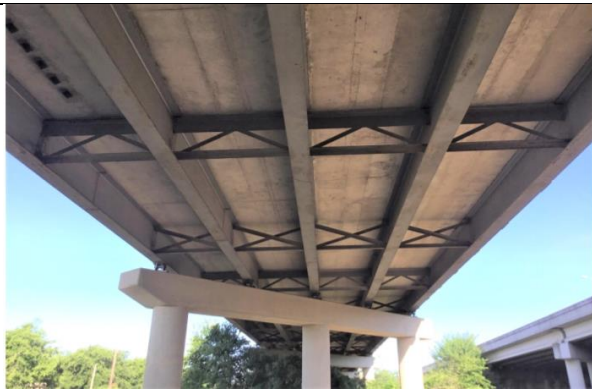
Superstructure (Looking West)
