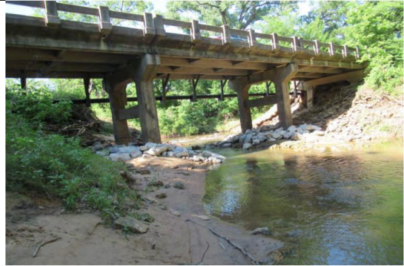
STREAM UNDER BRIDGE Looking Northeast
