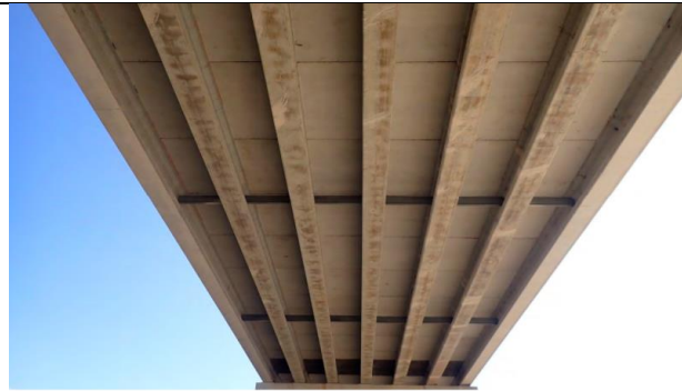
Underside of superstructure in Span 2 looking east.
