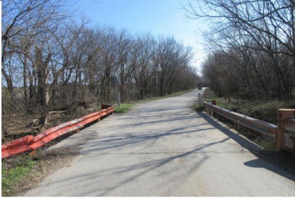
Roadway View Looking East
