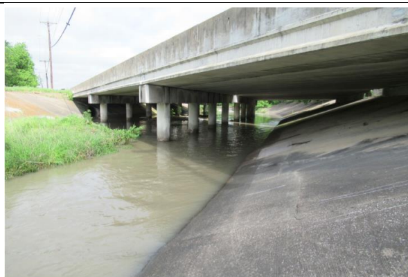
STREAM UNDER BRIDGE Looking Northwest
