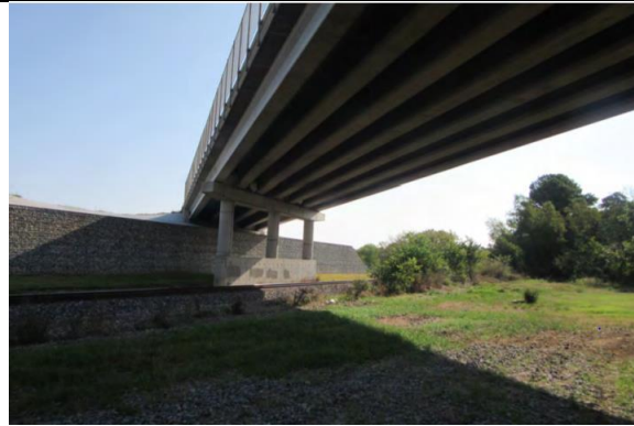
Up Rr Looking Southeast
