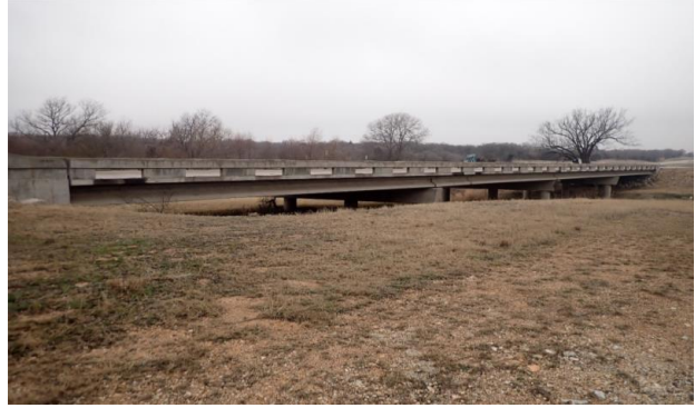
Northeast Bridge Elevation Looking West.
