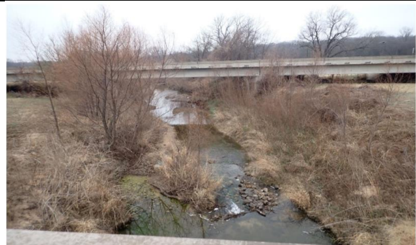
Downstream Channel Looking Southwest
