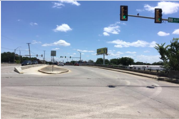
ROADWAY OVER BRIDGE - SYLVANIA AVENUE SOUTHBOUND (LOOKING SOUTHWEST)
