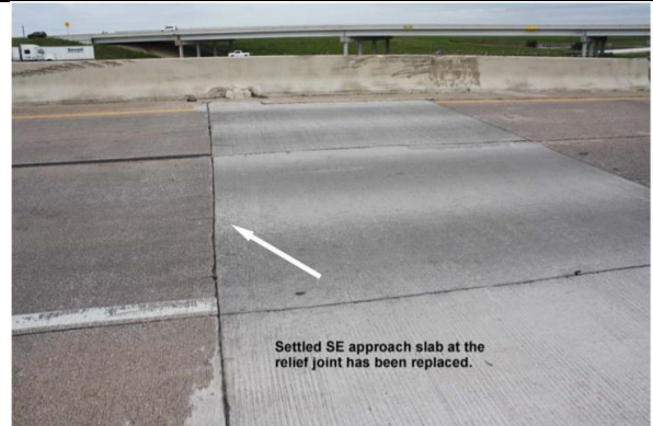
REPLACED SE APPROACH SLAB LOOKING NORTHEAST
