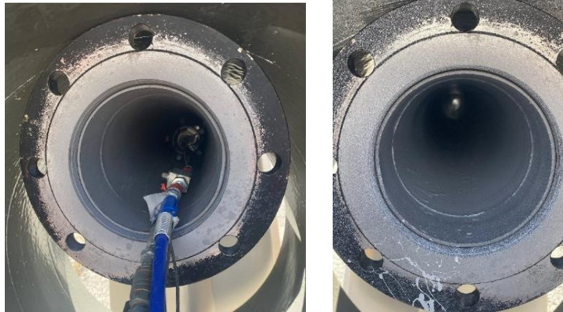
Figure 4.19 Inside View of Pipe After Primer Application
