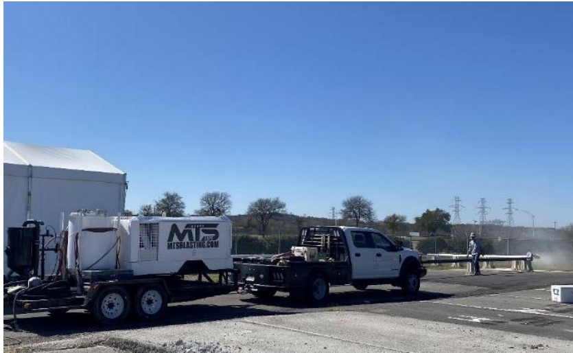
Figure 4.15 Sand Blasting in Progress
