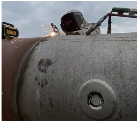
Figure 3.25 Pipe Sample 2 in. Hole Spanning
