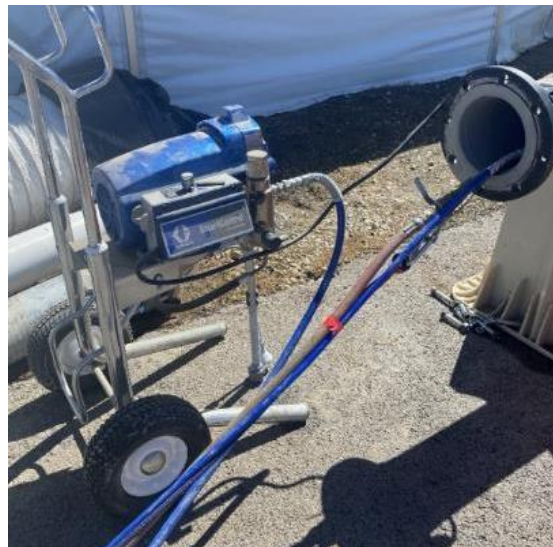
Figure 4.18 Primer Application in Progress
