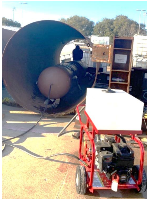
Figure 3.18 Complete Test Setup
