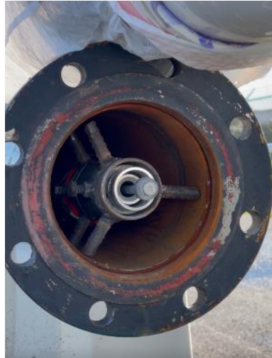
Figure 4.12 Inside View of Carbon Steel Pipe before Sand Blasting
