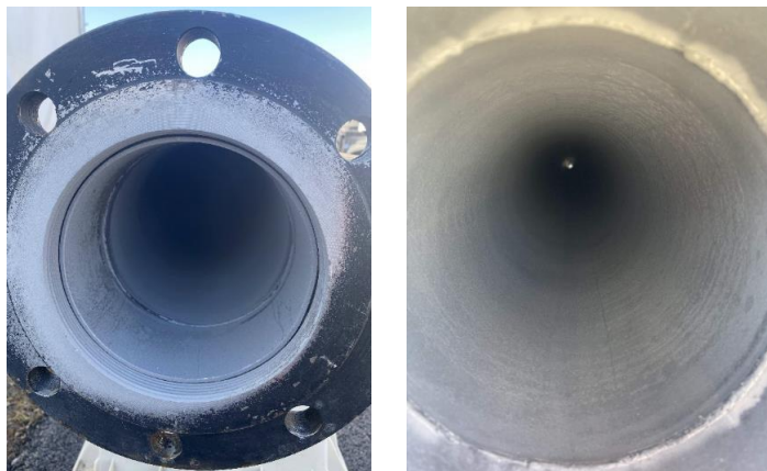
Figure 4.16 Inside View of Pipe After Sand Blasting
