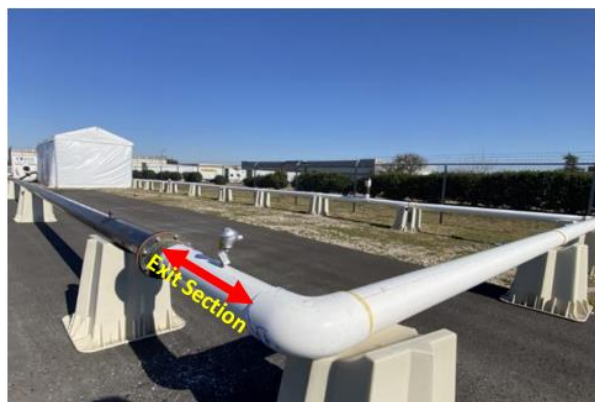
Figure 4.8 Thermocouple Installed at Exit Section
