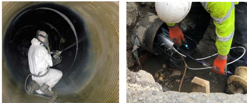
Figure 1.7 Larger Diameter Pipe Rehabilitation (Left) Source: CUIRE, and Smaller Diameter Pipe Rehabilitation (Right) Source: DrainsAid
