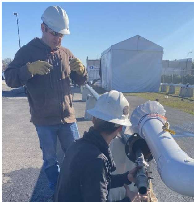
Figure 4.14 Sand Blasting Before Liner Application
