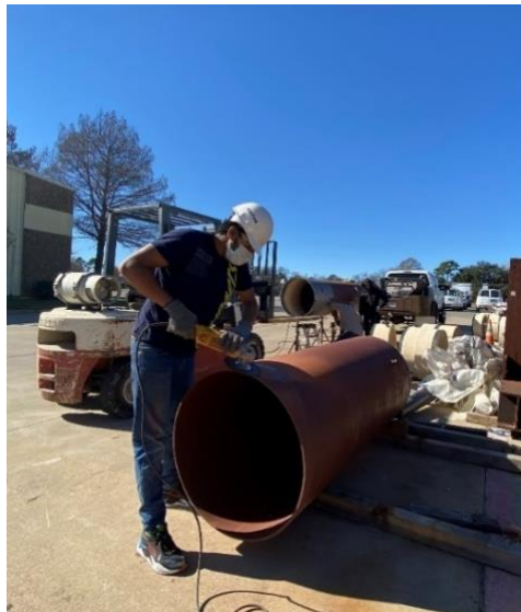
Figure 3.10 Spigot End Grinding before Welding
