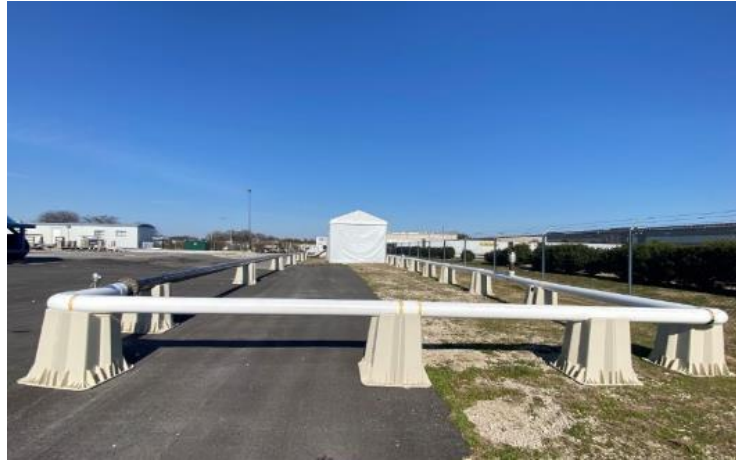
Figure 4.9 PVC Pipe Return Loop
