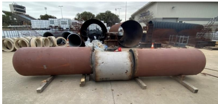
Figure 3.20 Cutting the Welding Joints from Spigot Ends to Separate Out the Middle Test Section
