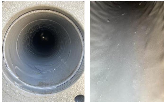
Figure 4.20 Inside View of Pipe After Liner Application
