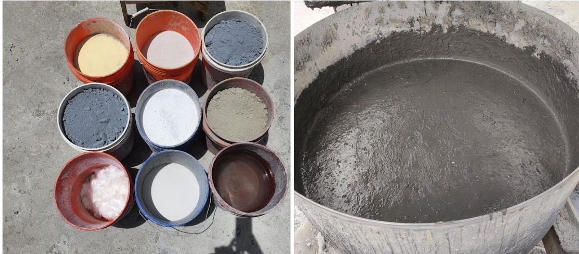
Figure 3-9 Material preparation and mixing
