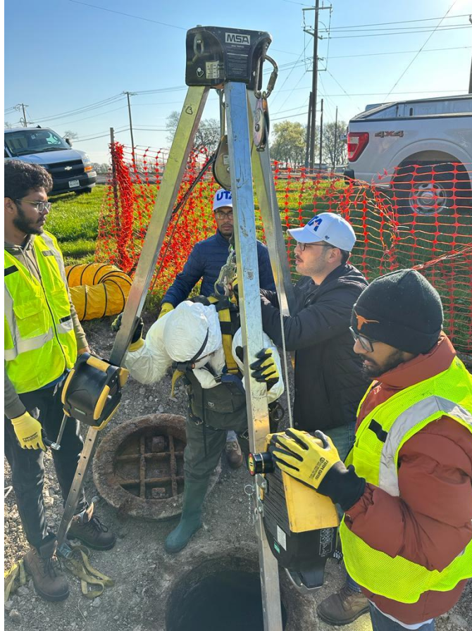
Figure 6-1 Confined space entry
