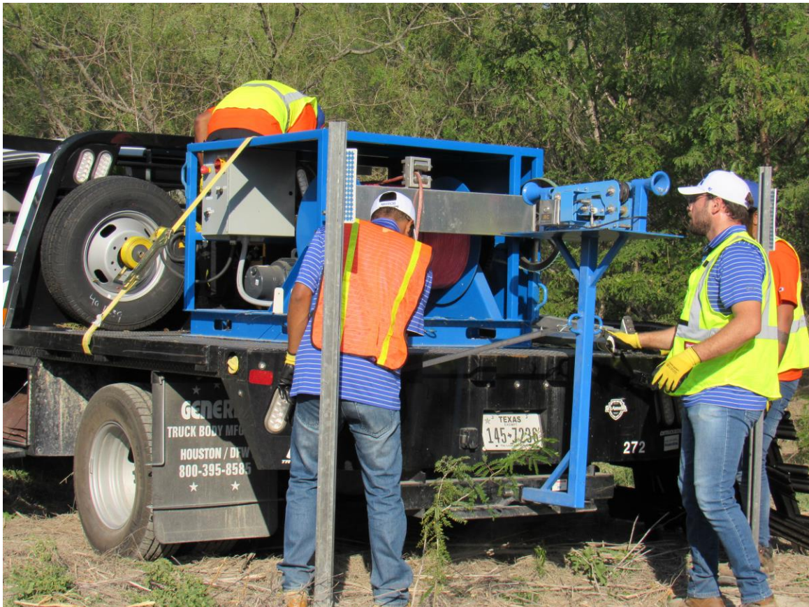
Figure 3-17 Cable winch and counter stand being operated.
