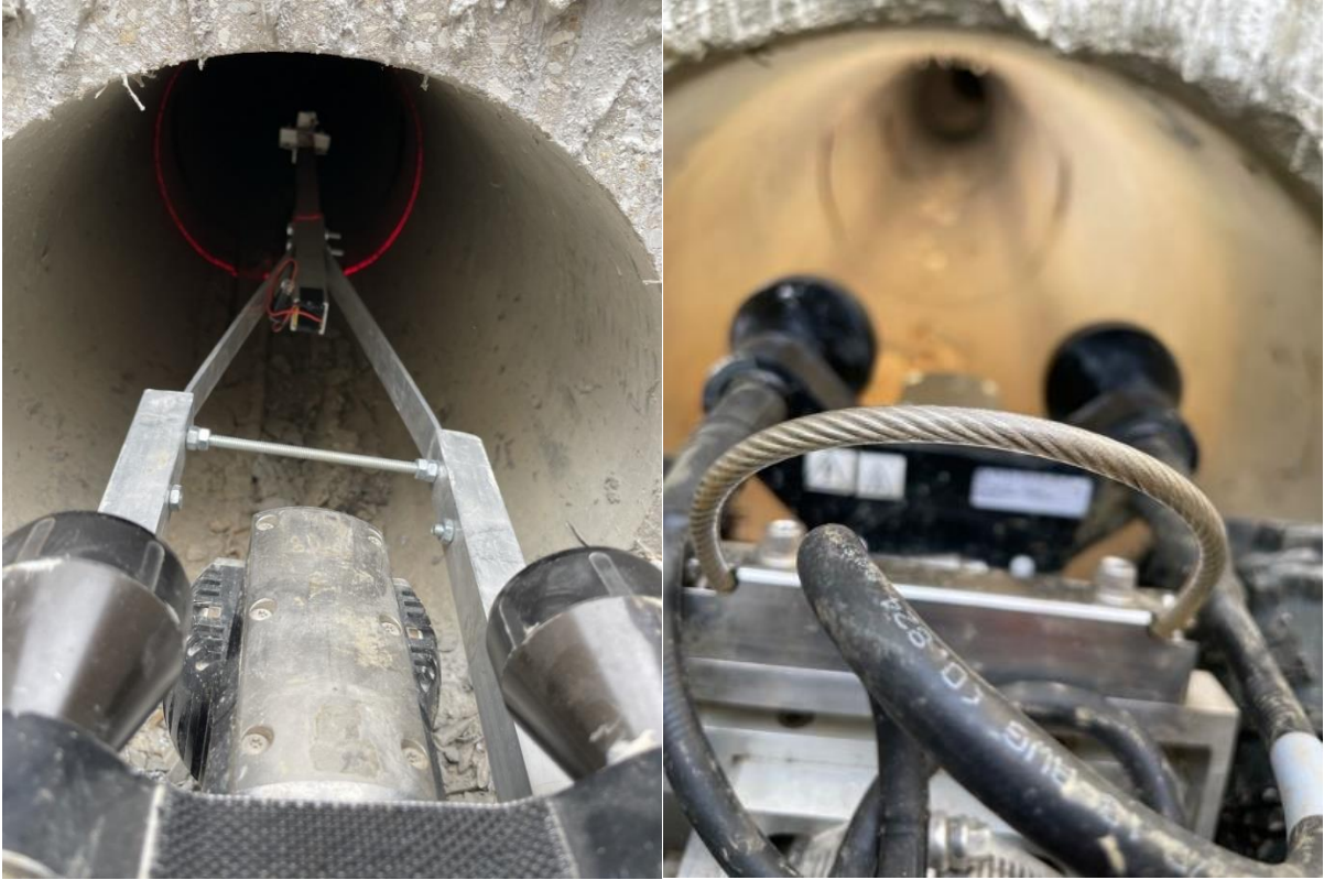
Figure 3-2 Crawler system utilizing CCTV and laser sensor.
