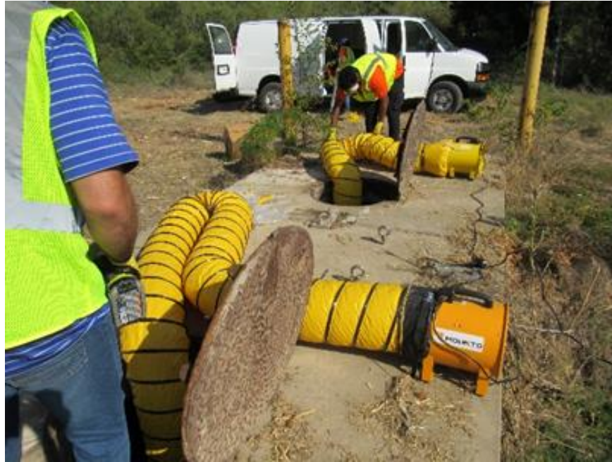
Figure 6-3 Air blower used prior to confined space entry
