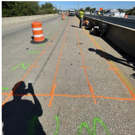
Figure 4- 16. GPR scanning on Lane 1S
