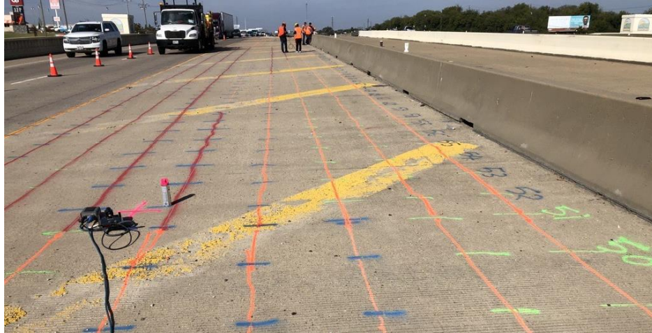
Figure 4- 19. scanning over the US-80 Bridge deck
