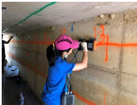
Figure 4- 14. The GPR scanning on the wall
