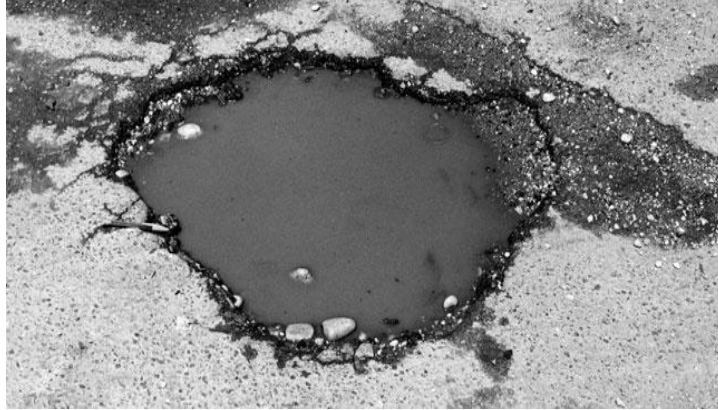
Figure 2.30 Moisture damage
