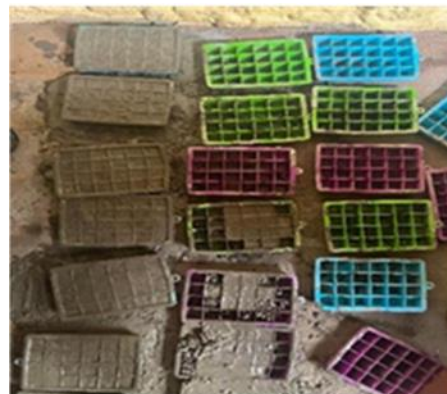
Figure 41. Concrete Cubes for Cover
