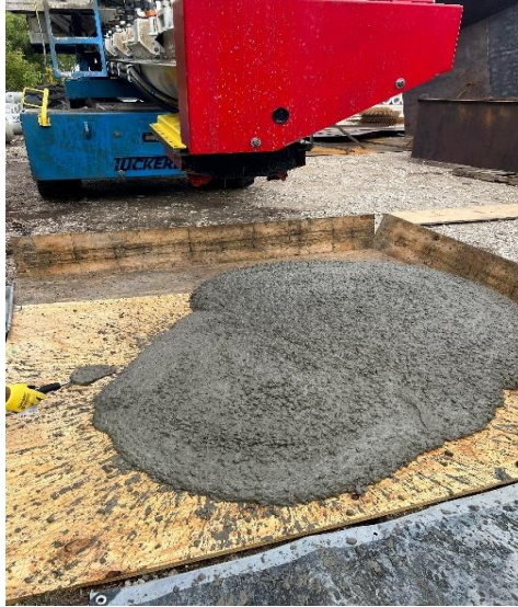
Figure 30. Concrete Provided at Forterra
