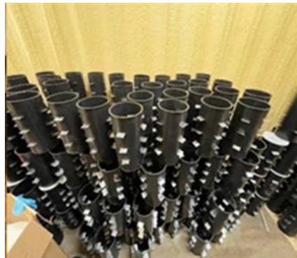
Figure 39. Placing the Spacers
