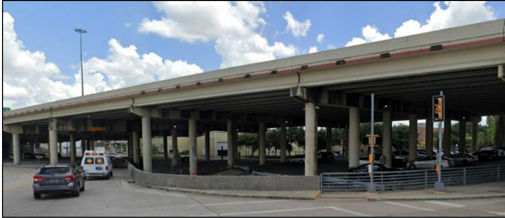
Figure 2.2. Horizontal openings on a bridge in Houston (Source: GoogleEarth, 2021)
