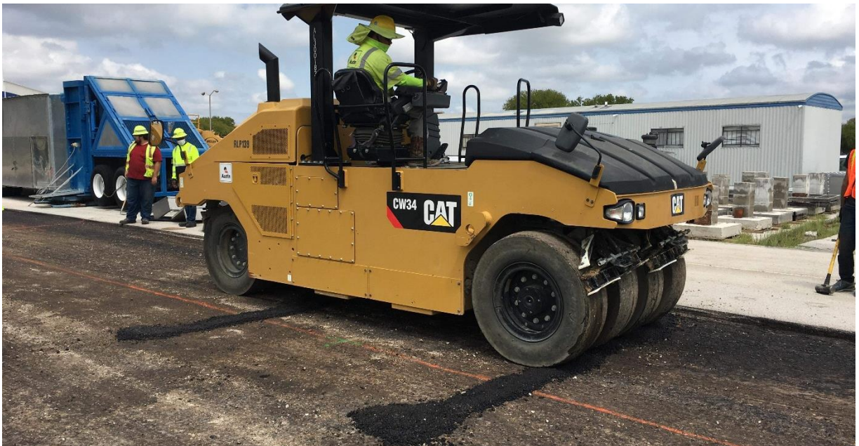
Figure 3.22 Instrumented sections M and N-ready to be paved
