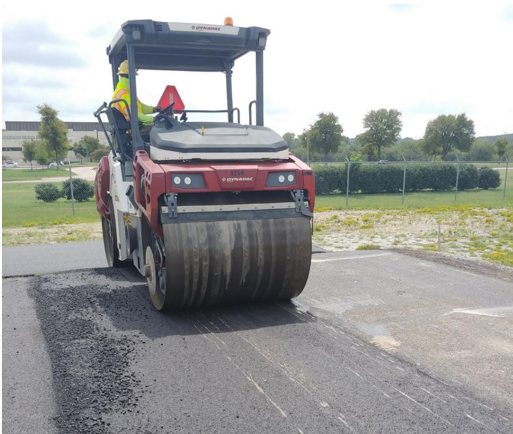
Figure 3.25 Steel Roller Compacting the Pavement HMA Sections
