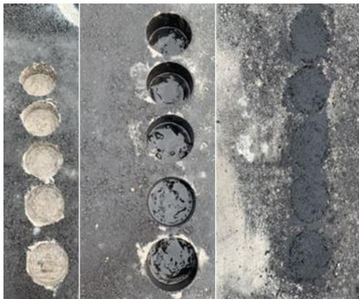
Figure 4.2 Sequence of covering the core holes
