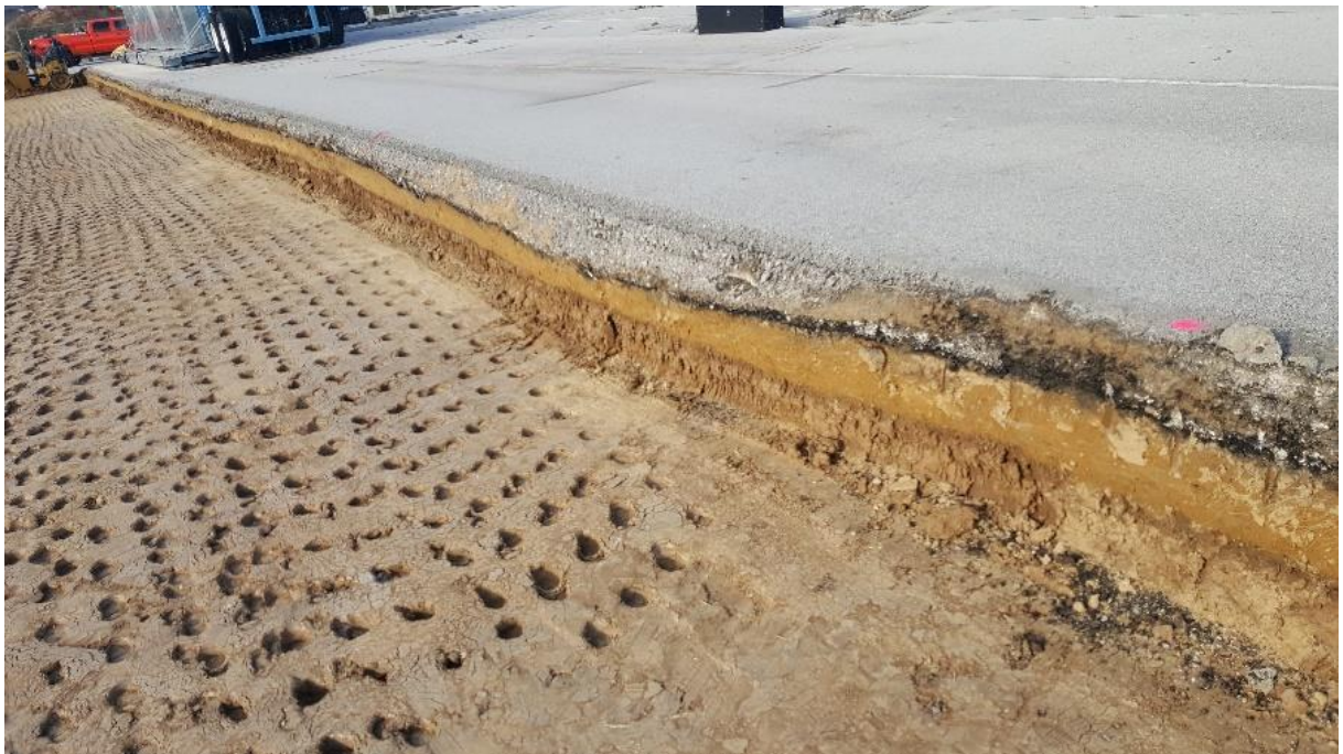
Figure 3.10 Compaction of new subgrade soil
