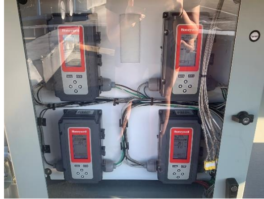
3.6 Electrical box equipped with data logger
