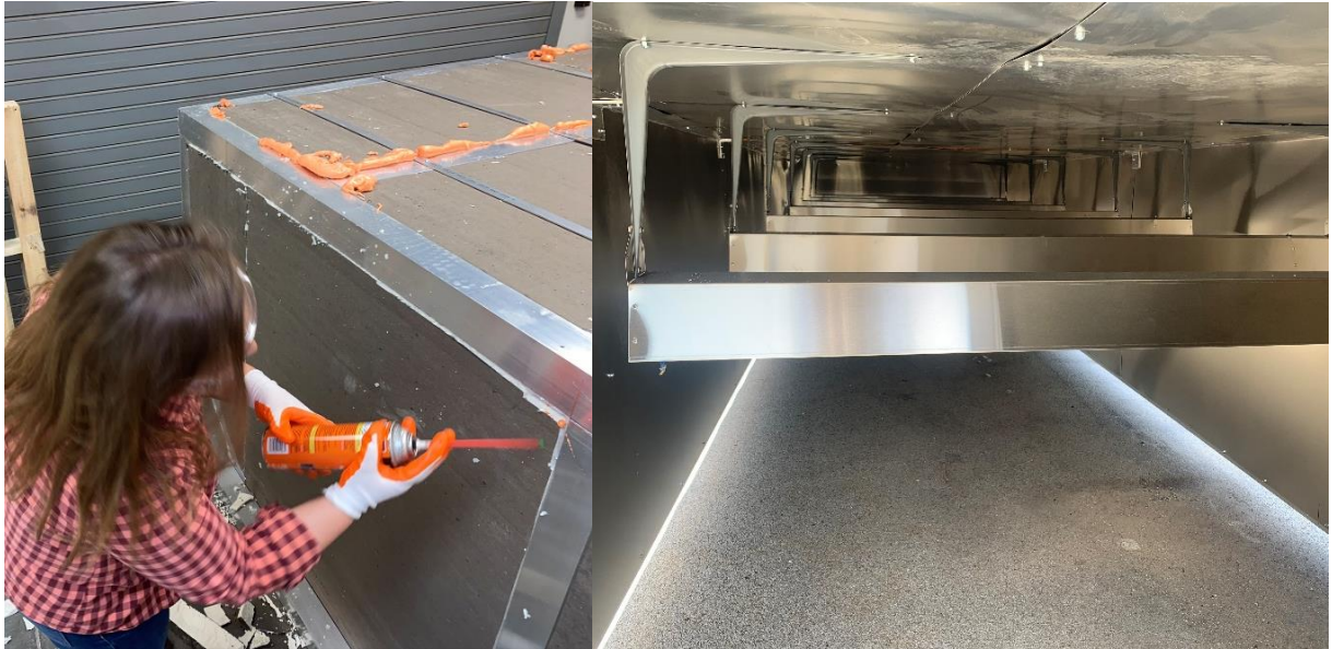
Figure 3.5 Construction of the oxidation chambers
