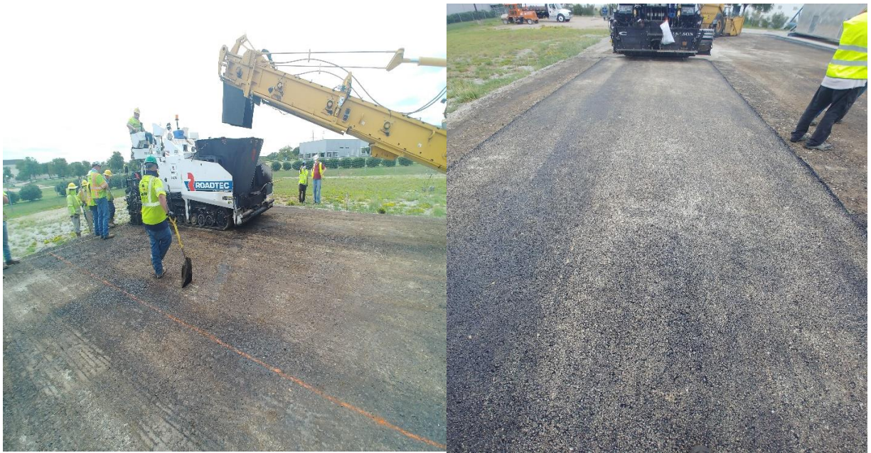
Figure A4-1 Paving of Section P
