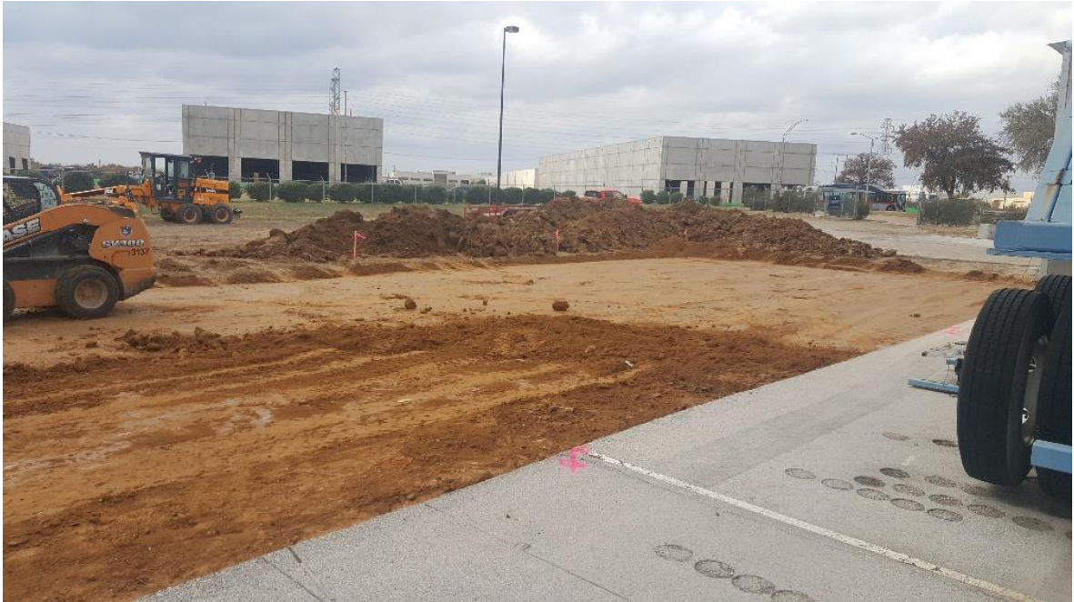
Figure 3.9 Placement of new subgrade soil
