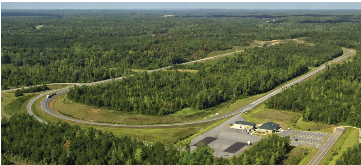
Figure 2.18 NCAT Test Track – Alabama
