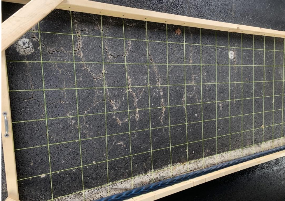
Figure 3.62. Crack extent evaluation using a grid panel of squares
