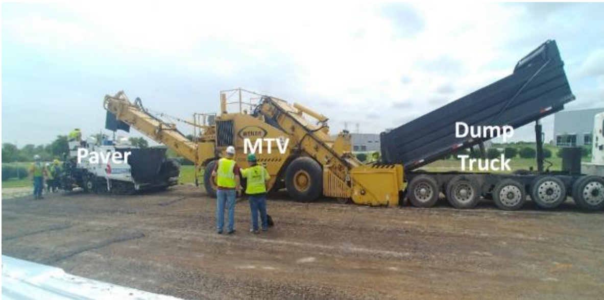
Figure 3.24 Sequence of Asphalt Mix Paving
