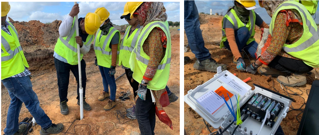
Figure 3.10 Installation of the sensors at Parks Springs site
