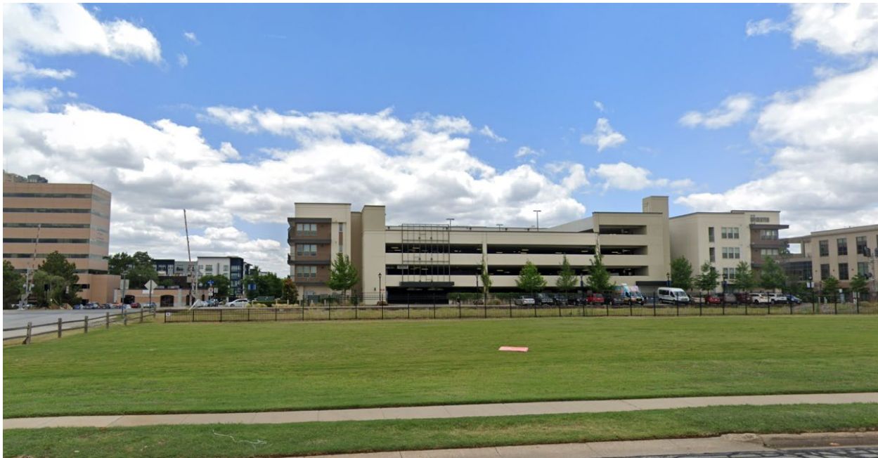
Figure 45 Existing Condition of Civic Plaza (Source: Google Maps)
