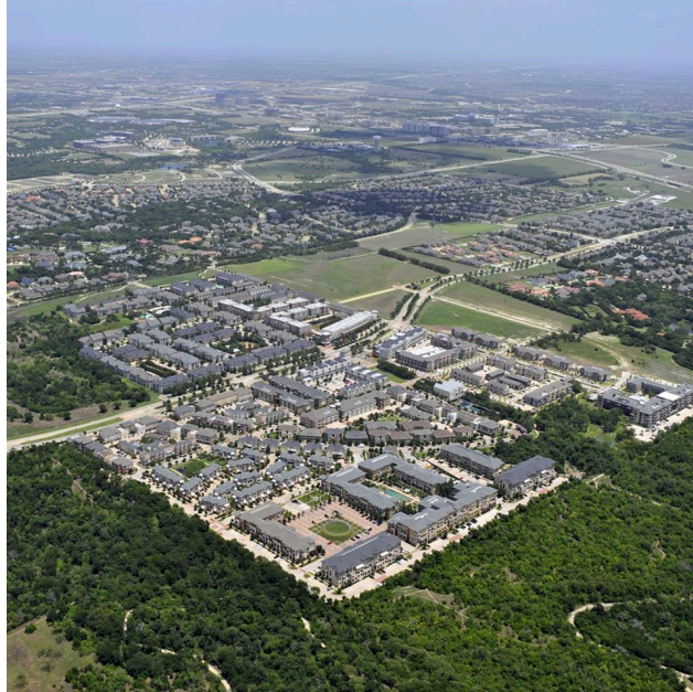
Figure 4. 16 Austin ranch aerial, Source: Thousand Oaks at Austin Ranch, 2017
