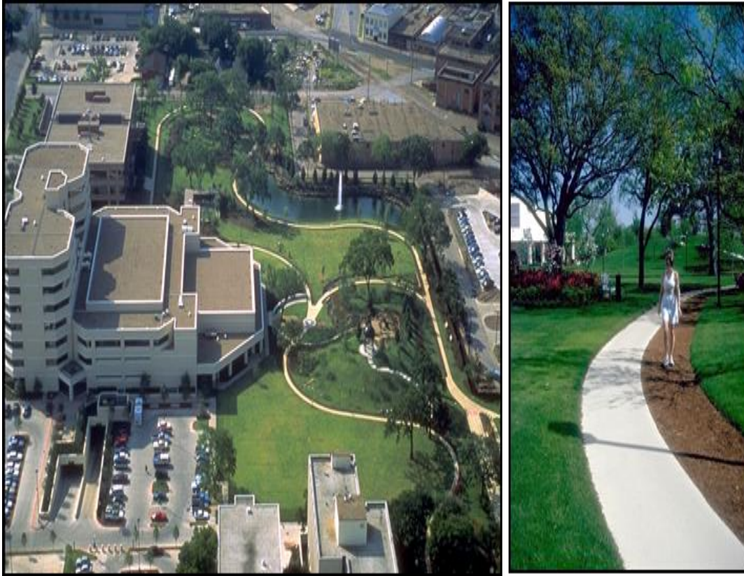
Figure 0-13 Baylor University Medical Center's Tom Landry Fitness Park – “This wonderful 7.5 acre fitness park is on Baylor's Downtown Dallas Campus was created partly, by using the soil excavation to create a small pond and water feature and a large hill named 'Victory Hill', complete with a classically designed shade structure, sculpture, quiet spring near a sitting area, that ran from the gazebo, cascading down to the 'Warm-up Circle' and a good vista from the fitness center's natatorium. The hill celebrated the hospital's cancer patients that won a victory at the near-by cancer center. The Fitness Trail was designed for ½ and a full mile track that ran through classic formed 'outdoor rooms' with selected views planned to the Dallas Downtown Skyline, and special plantings to provide visual interest when exercising”(Source: Rowland Jackson, 2016).
