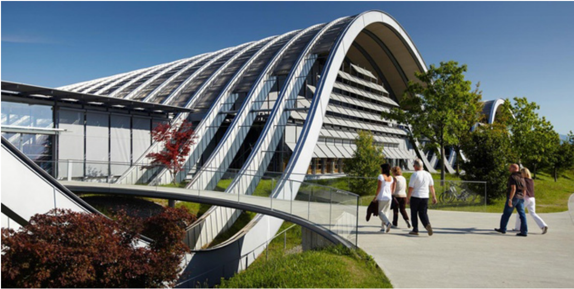
Figure: 2.5.4: Zentrum Paul Klee, Berne, Switzerland, Architect: Renzo Piano (Source: designrulz, 2017)
