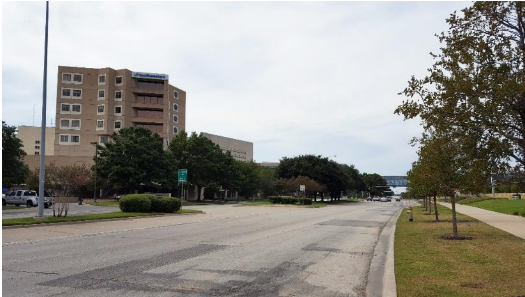
Figure 3-7 SWMD; Harry Hines Boulevard
