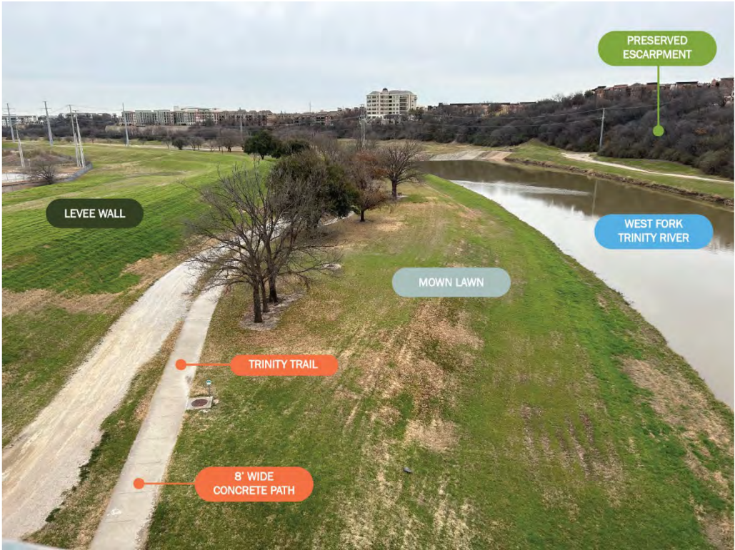
Figure 42 Northern Levee Looking Down from North Main Street Bridge (Adapted with Illustrator)
