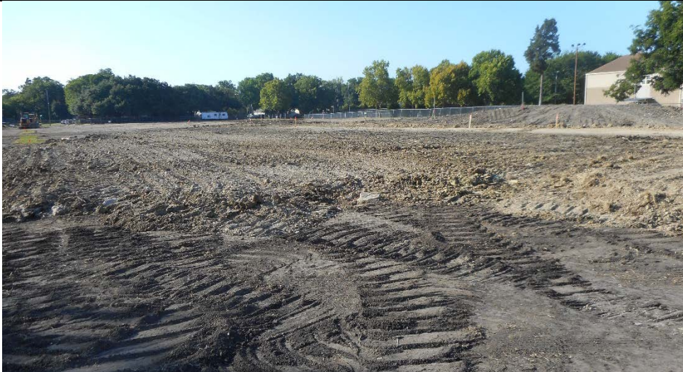
Figure 6. Removal of vegetation. Park construction site in Dallas, Texas.
