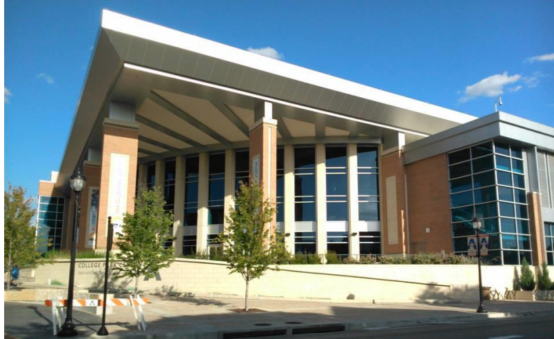
Figure 4-55 College Park Center on campus
