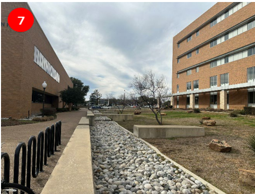
Figure 5-12 View to Cooper & Parking Lot
