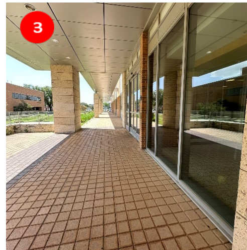
Figure 5-8 Windows at ERB: No Seating
