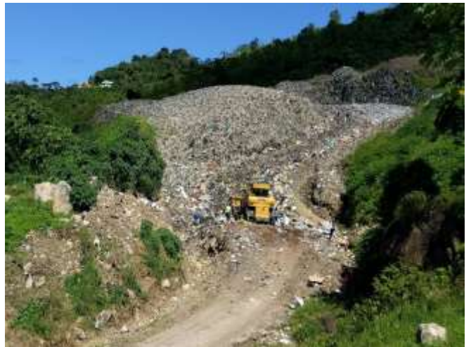
Figure 2.7. Track loader operation
