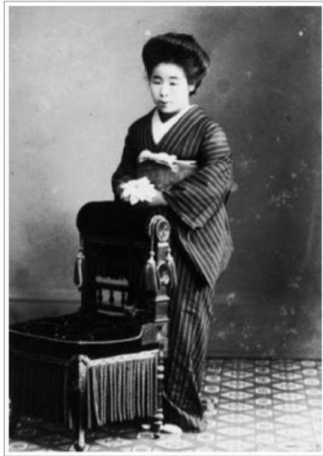
Figure 2.2: Kaku Kono's exchange photograph, 1920. Retrieved from Kawakami's Picture Bride Stories
