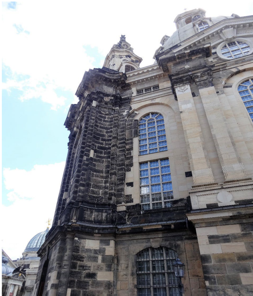
Figure A.2: Side view of the Frauenkirche, showing the patchwork of old and new stones (courtesy of the author)
