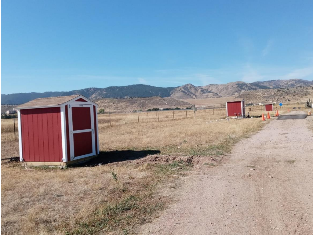
Figure 3: View of METEC Urban testbed showing Structure1 (Concrete slab foundation), Structure2 (Basement), Structure3(Crawlspace), the road running through the testbed and the Asphalt pavement in front of Structure2.
