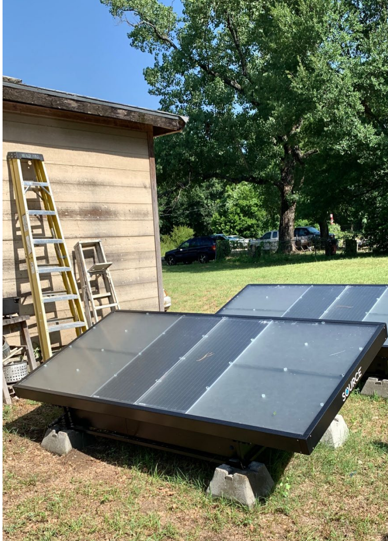
Figure 4.1: Fully installed SOURCE Hydropanels in a resident's backyard, bringing potable drinking water straight to their kitchens through minor plumbing. Note: Perez Vela, J. (n.d.)
